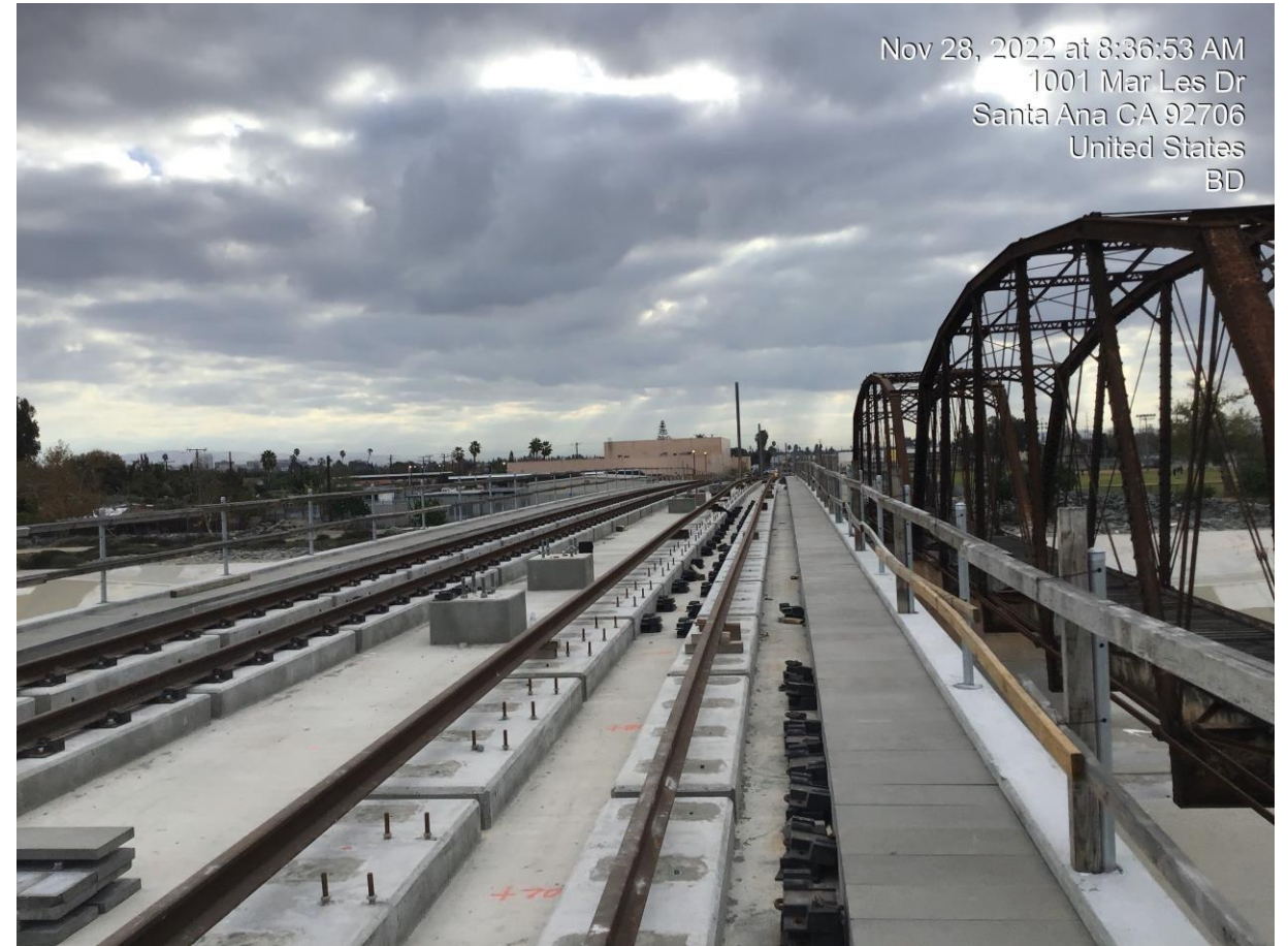
Santa Ana River Bridge Plinths
