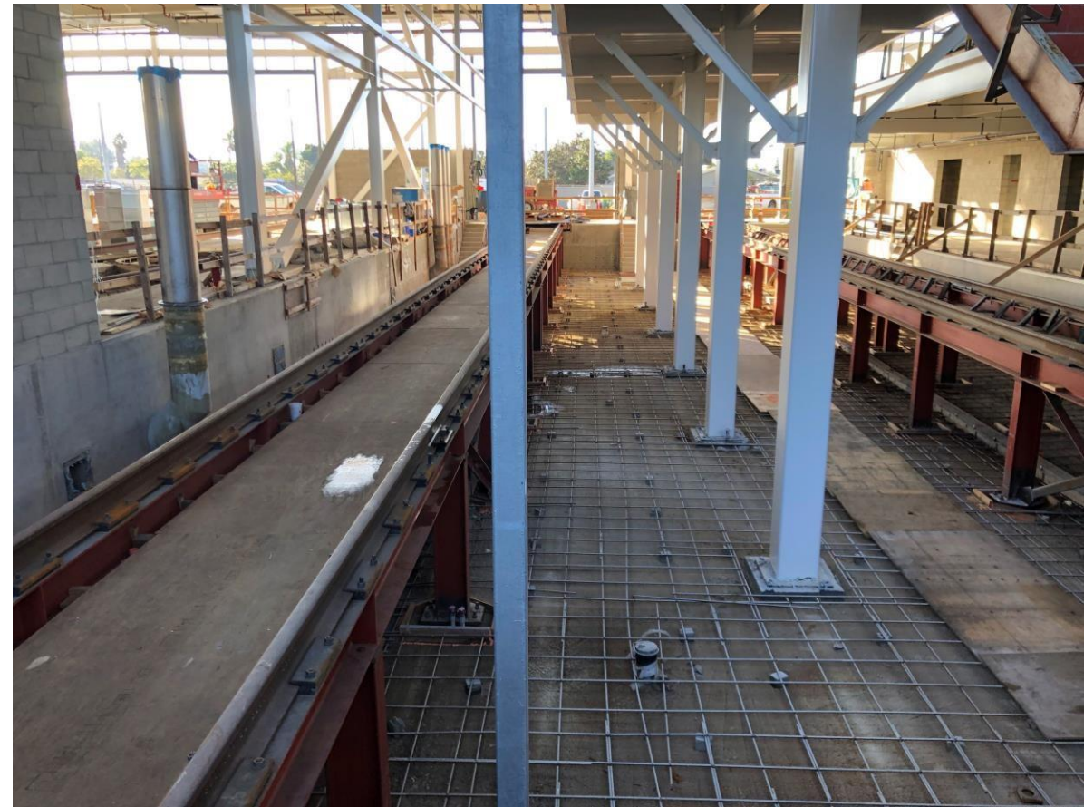
Tracks within the Service and Inspection Pit
