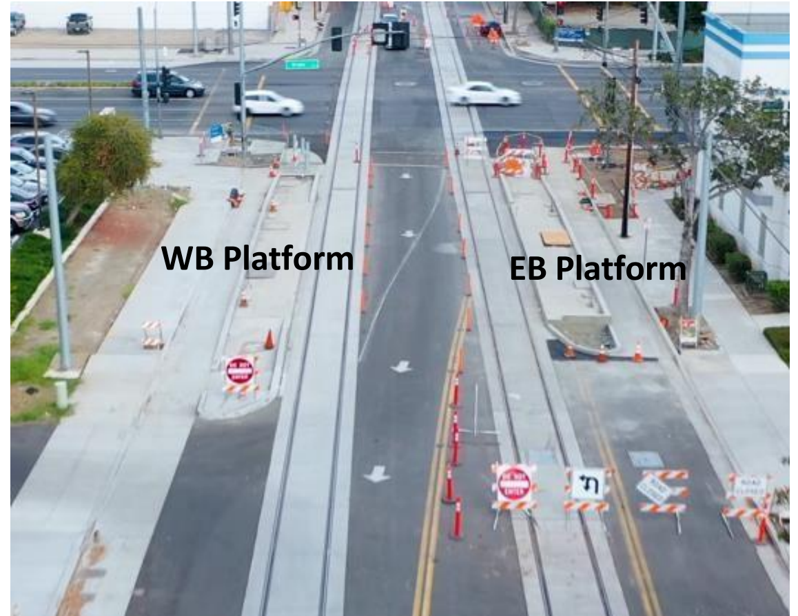
Bristol Side Station Platforms
